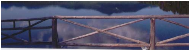
Current Bridge Railing
