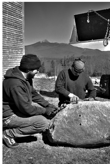
From left: Stonemason Gary Jones in front of the in-progress Basin View Lot wall; Eric Dube and Pat Shea set feathers and wedges in a boulder. / Photos by Juno Lamb
